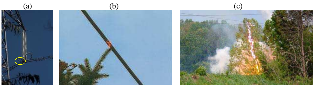
Figure 3. Images showing an example of electric poles, electric discharge, and fire ignition. (a) Detail of a cable joint/coupling; (b) example of air ionization caused by the proximity of a tree branch; (c) fire ignition caused by an electric discharge.
