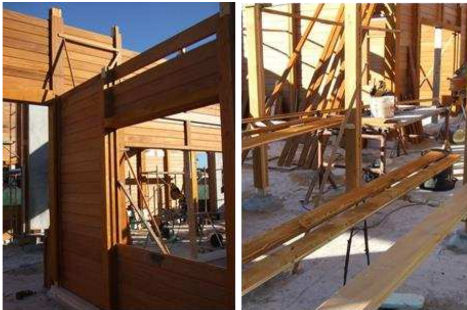
Figure 1. Wood-framed house under construction
