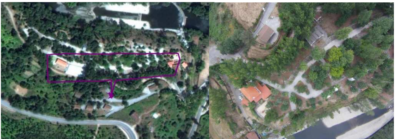
Figure 2. Left: Trajectory described by the quadcopter while on autonomous navigation over the area of the CP of Coja (seen on Google Earth). Right: One of the pictures taken during the flight with a GoPro camera.
