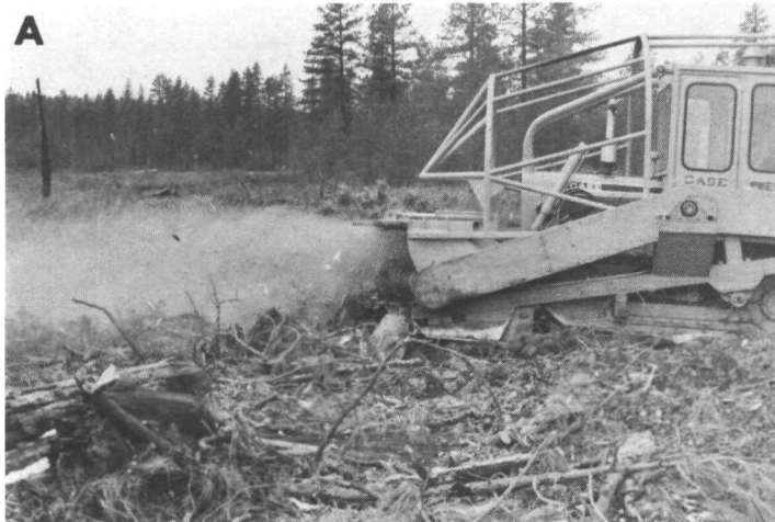
Figure 3.--Tree Eater operation on Deschutes National Forest: A, Treating logging residue prior to planting seedlings: B, appearance of residue after treatment.
