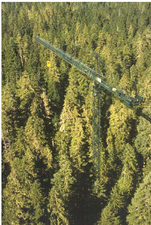
FIG. 17.3 Canopy cranes are a relatively new tool for experimental access to forest canopies. For example, the gondola of the Wind River Canopy Crane (75 m tall tower, 84 m long jib) can access 700,000 m 3 of 60 m tall canopy, as well as the canopy–atmosphere interface, over a 2.3 ha area in a 500-yr-old Pseudotsuga/Tsuga forest in southwestern Washington, U.S. Photo by J.F. Franklin, Reprinted from D. Shaw, (2004) with permission from Elsevier.
