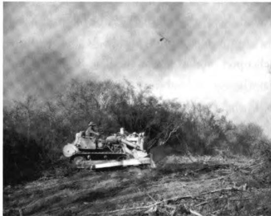
Bulldozer building fire line, Wheeler Springs Fire, Los Padres National Forest, 1948. By this time, bulldozers were a key factor in fire line construction in Region 5.
